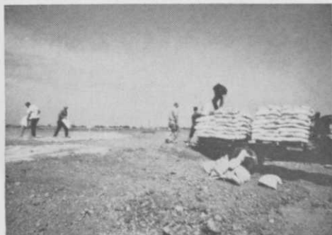
Turface is dumped with fill dirt in a proportion of about 1 to 3.
