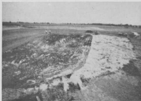
After topsoil has been laid, additional Turface is worked in by discing.
