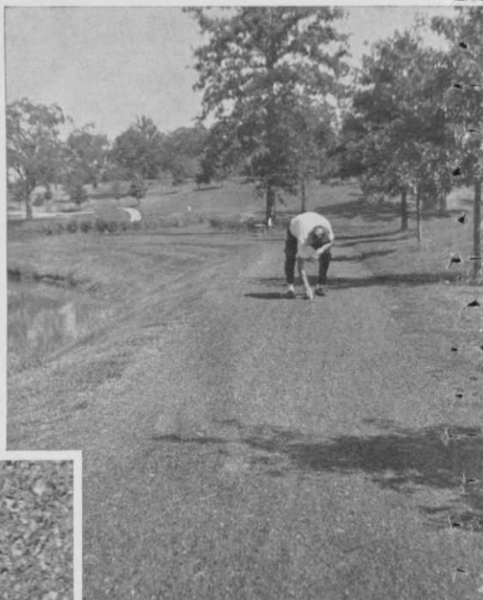
Here is one of the pecan shell car paths at the Old Warson club in St. Louis. Inset photo shows surface and slight decomposition of buried shells.
