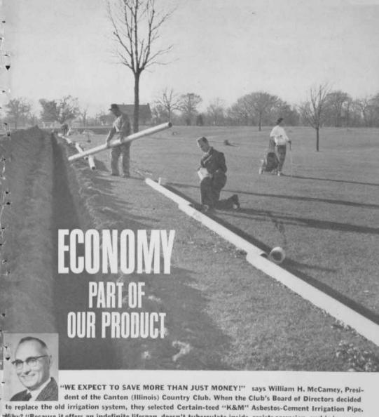
Why? "Because it offers an indefinite lifespan, doesn't tuberculate inside, resists corrosion, and is immune to electrolysis and ground acids," Mr. McCamey points out. The club saved approximately 20% in initial material costs, compared with metal pipe. Installation was fast and economical, scarcely noticed by many golfers. Now, further savings lie ahead-in time and maintenance.
