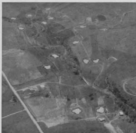
Greens in this aerial photo of the Sooner course in Bartlesville, Okla., show in white because Architect Floyd Farley specified limestone chips on the sub-grade as part of the drainage plan. Unusual photo was made by D. S. Willcox before topsoil was brought in.
