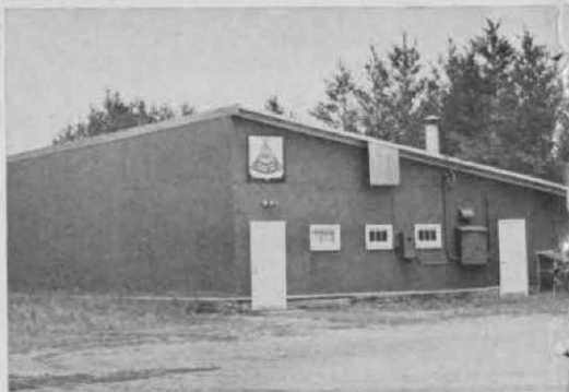
Two-sheet, pole building structure that cost $22,500 to erect is operated by the Stevens Point (Wis.) CC. Building can be expanded so that two more curling sheets can be added. Present ice making equipment will handle four sheets. Building is 170 x 30 feet.
