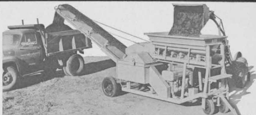
The versatile "L" machines shred and then load from conveniently high discharge levels—popular with Golf Course Builders, Architects, and Supts.
