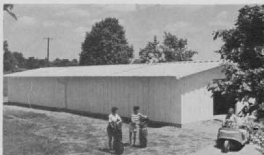
Garage accommodates 36 cars and can be expanded, if necessary. It cost less than $5,000 to erect this structure.
