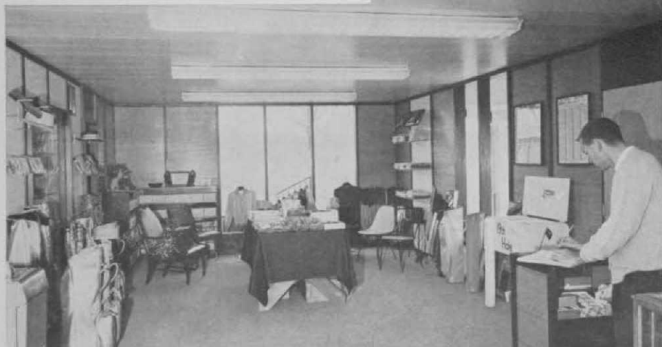
Steel pro shop at Brown's Run is 28 feet wide and 44 feet long, was selected by architect because it is easily maintained. Interior walls are finished in wood panelling.
