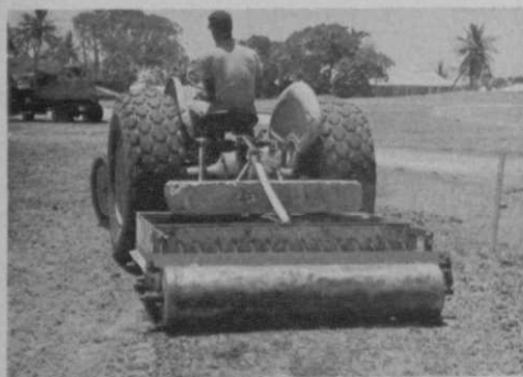
Close up view of cutting discs and roller.
