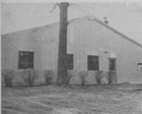
Pre-fab steel building at North Shore was built in 1957, is divided into three large sections.
