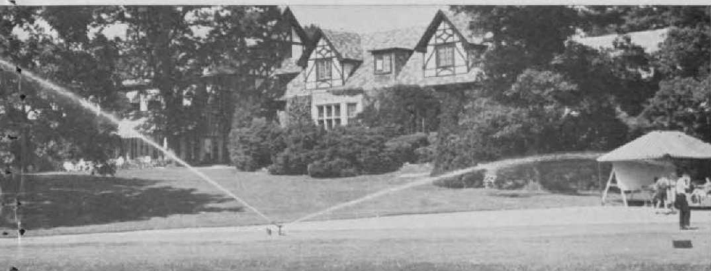
Practice green at Butterfield with typical irrigation sprinkler head operating. Butterfield uses cast iron mains exclusively to water its grounds.
