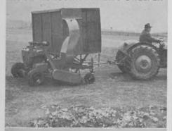
Leaves are everybody's problem! For fast, efficient removal of debris, and wet or dry leaves use a towed B-25 Mulch-Vac which can cover more area more efficiently than men using other methods. The debris will be collected by the Mulch-Vac, mulched, and then deposited in a four cubic yard cage attachment. If desired, leaves can be vacuumed, mulched and then automatically respread as natural fertilizer.
