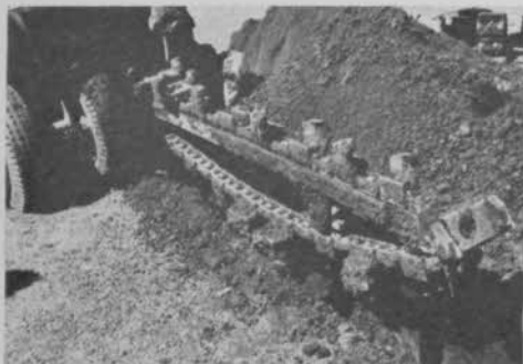
Digging mechanism on the power digger.
