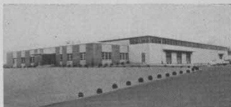
Consolidated Pipe's new plant in Stow, O.
