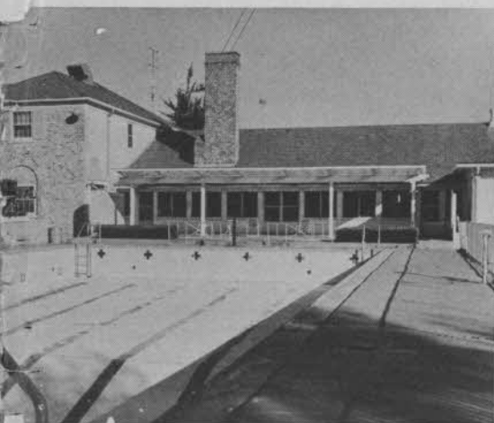
Swimming pool (above) was built about five years ago. At right is a view of one corner of the large lounge. Westbrook's clubhouse is re-decorated and refurnished about every five years.
