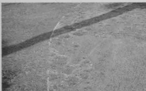
Bermuda grows right back through the blacktop if excavation is shallow.
