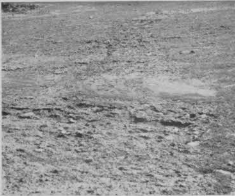
Unchecked erosion on newly planted fairway is costly, unsightly. This is minor damage compared to some.
