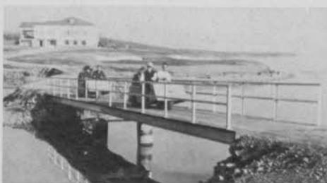
The aluminum bridge in the foreground and the one directly behind it carry golf cars and golfers across a lake inlet at the Turtle Point Yacht and CC in Florence, Ala. The bridges were designed and fabricated by Reynolds Metal Co., and were erected with hand tools in only two days. In the background are the 9th hole, clubhouse and a view of the Tennessee River. The bridges have a 5,000 lb. plus capacity and were made at Reynold's Phoenix, Ariz., plant.
