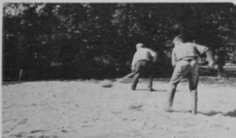
Mixture is leveled with rakes turned upside down.
