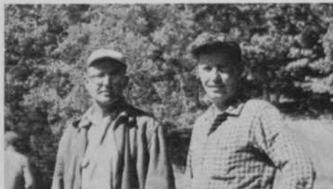
Ted Newville (l) and Maynard Erickson were in charge of the Wirth Park construction job.
