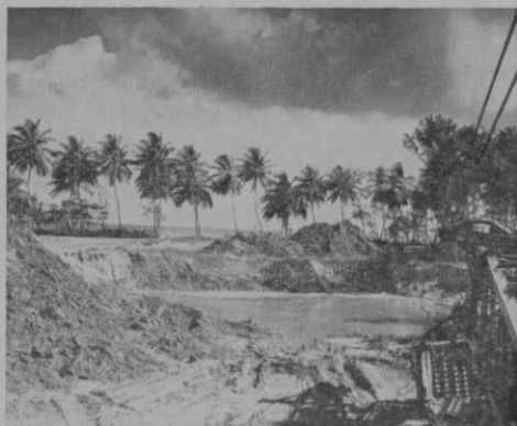
Construction of the 9-hole extension of the 18-hole Dorado Beach GC, Puerto Rico, started last January, will be completed soon. The new 9 begins and ends in the vicinity of the clubhouse.
