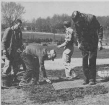
Steel mat is placed on stolons and firmed under foot to press them into soil.
