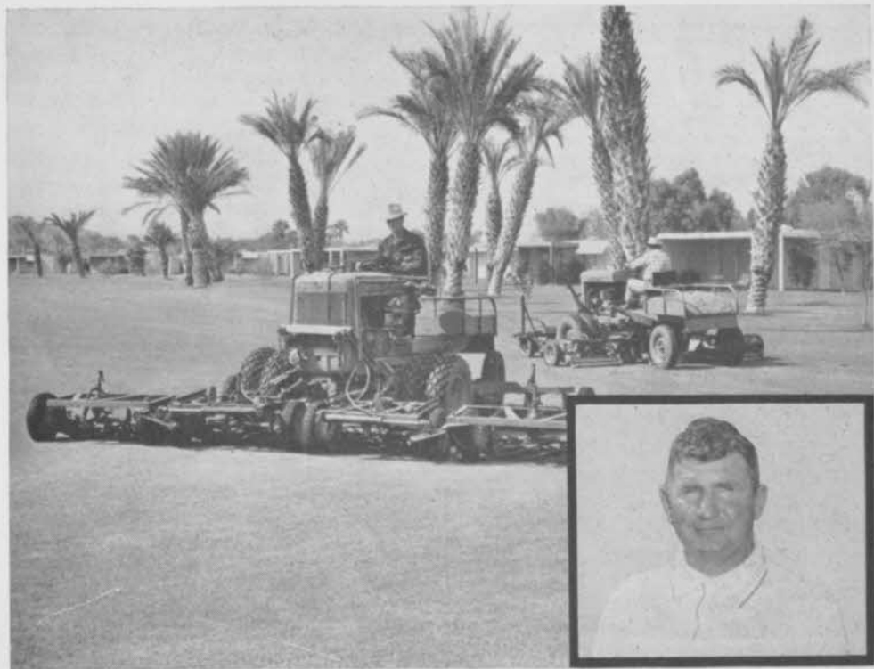
Jacobsen-Worthington Model "F" Tractors with seven gang and five gang mower units.
