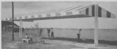
framework of alloy steel that it recommends for driving ranges. The canopy has a 9-or 12-in. fascia for advertising purposes and can be obtained in a combination encompassing a choice of 12 colors. The Kar Kover is of all nut and bolt construction, is built to withstand 90 mph winds and supports a roof load of from 3 to 5-ft. of freshly fallen snow. Water runs off quickly and freely from both sides.
