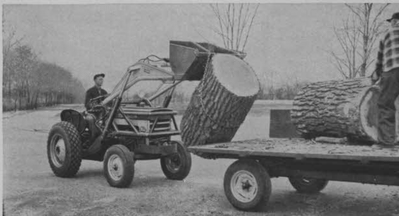
38.5 hp* International 240 Utility tractor with International Wagner loader.
