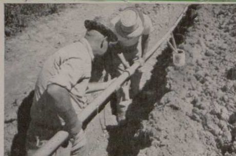
Joining Uscolite pipe with UscoWeld* solvent-weld fittings. Each joint takes about 90 seconds to make up and is locked for life.
