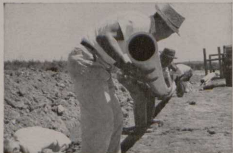
Laying 6" Uscolite pipe in Pine Ridge Golf Course. Despite its size, this 40' length is easily handled by three men.
