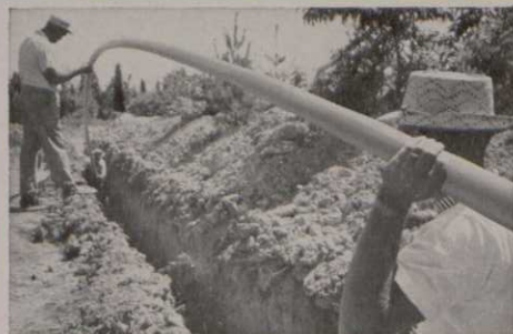
Note the flexibility and easy handling of Uscolite pipe, being placed in a 3-ft. ditch.
