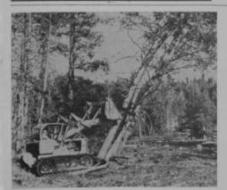
International Harvester's Drott TD-20 Four-in-One uses its bucket to topple trees on site of Meadowvale GC, near Lake Tahoe. The Drott removes 200 trees daily and piles them for burning. Designed by Bill Bell, Pasadena architect, Meadowvale's fairways will cross and re-cross Truckee river five times,
