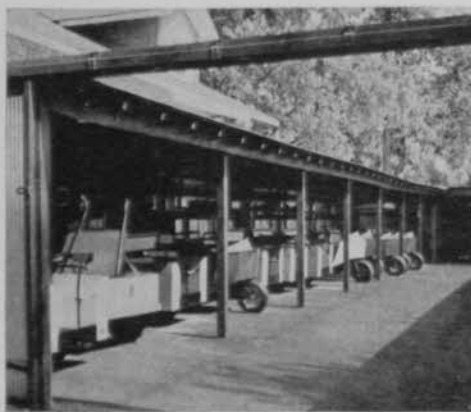
Garage at Idlewild CC, Flossmoor, Ill. is of a square U design with 12-ft. center aisle and sliding security door. Area is lighted at night to discourage theft or vandalism.
