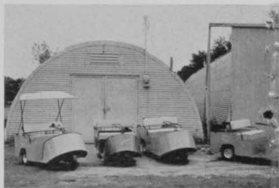
Quonset type garage houses cars at the Country Club of Lincoln, Neb. It is made of aluminum sheeting and is located next to club's maintenance building.
