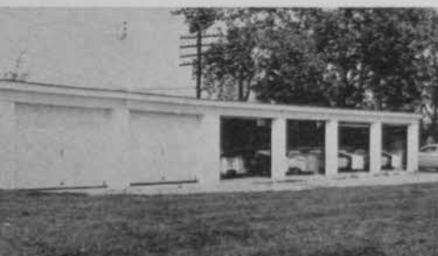
Garage at Olympia Fields is of concrete block, one of three at club. Members paid $350 per stall to underwrite construction. They pay $20 per month for maintenance and electricity.
