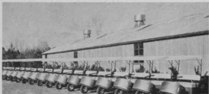
Utility type building at Lakeside CC, Houston, Tex., is constructed of galvanized sheeting. It has large capacity, is quickly expandable.
