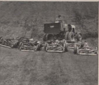
FAIRWAYS? 7-unit Universal Frame (shown with Toro General Tractor) mows a swath 13 ft. wide.
