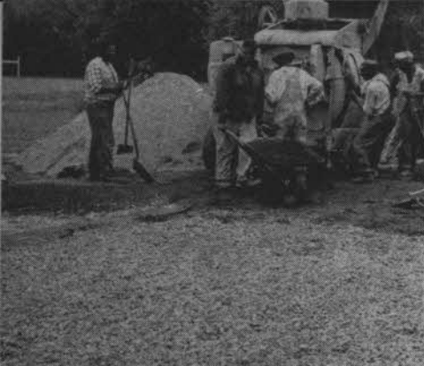
Danner supervised building of three bent greens at Belle Meade, also in Nashville. In foreground is gravel sub base; at rear topsoil is being mixed.
