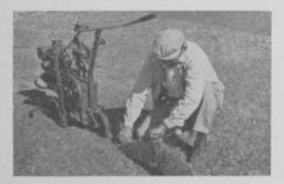
Lay-over feature of Ryan trenching blade leaves sod undamaged, permits neat, easy replacement,
