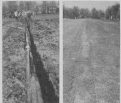
Left: 4-in. mechanical joint cast iron pipe being installed at Ridge CC, Right: One week after pipe was installed fairway was in excellent shape. You have to look hard to see where ground was excavated.
