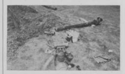
45 deg. bend was made and a sprinkler head installed at this point.
