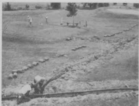
Pipe leading to a green and a tee was installed without interrupting play.
