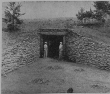
Gatlinburg's steep elevations are a treat for eyes but tough to tread. This tunnel between the 9th green and 10th tee makes the going easy.
