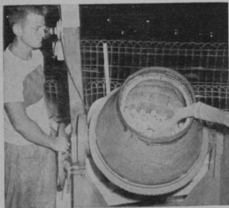
Sump pump feeds cleaning solution into brush lined mixer after quick loading thru open end.
