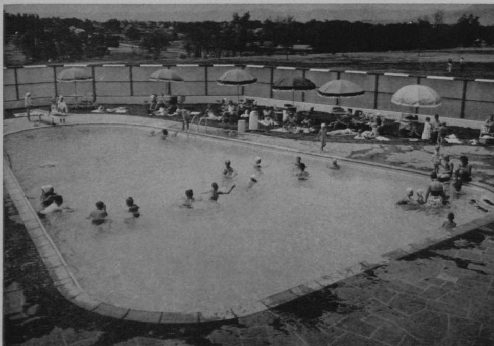
Lakewood CC, Denver Colo., pool is painted with the chlorinated natural-rubber-base type paint Ramuc because it has high resistance to penetration of pool water.
