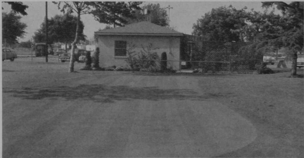
Starter house (20x30 ft.) at Southgate, Calif. course is also used by three recreation workers as their headquarters. Starter house is also snack bar. More than 60 clubs and about 12 dozen golf balls are stocked for rental purposes. One of the three practice putting greens is in the foreground. Southgate has three putting greens. Cups and flags are removed to indicate the green out of play.
