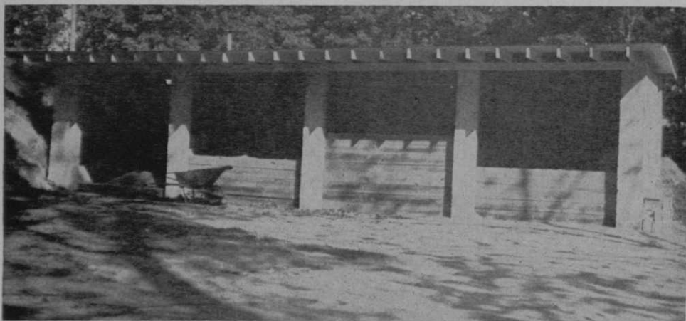
Back of the soil processing building, showing the four compartments for processed soil.
