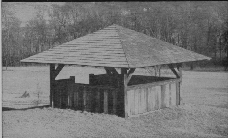
A Koppers Shelter House recently installed at the Oakmont Country Club, Oakmont, Pa.
