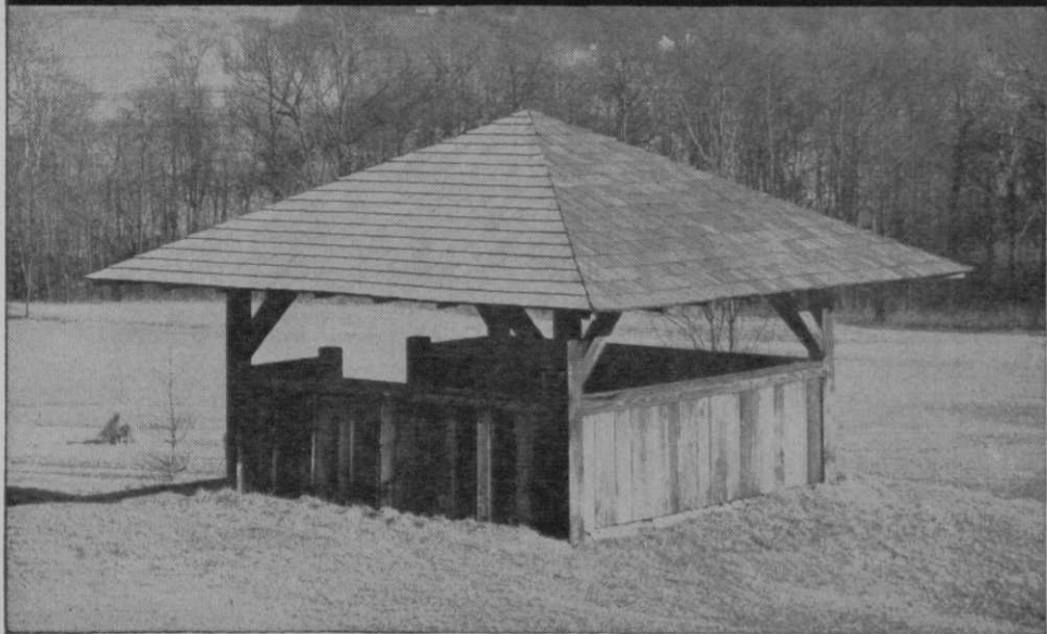
A Koppers Shelter House recently installed at the Oakmont Country Club, Oakmont, Pa.
