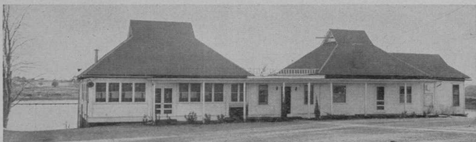
This beautiful little clubhouse between a lake and the first tee, was built from a dirty, dilapidated old structure.
