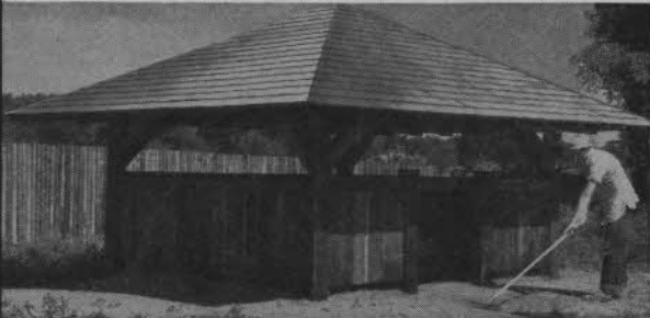
One of five Koppers Pre-Cut Shelter Houses recently installed at Oakmont Country Club, Oakmont, Pa.
