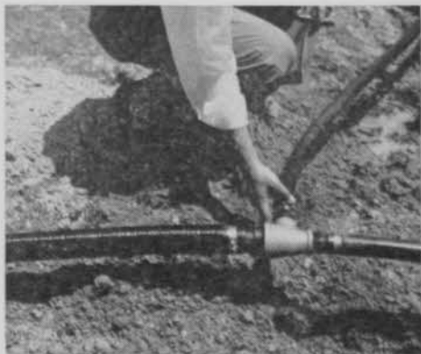
A screwdriver and hack-saw are only tools needed for installation of plastic pipe.
