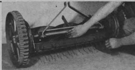
Flexi-combs fit Toro and Worthington mowers . . . Simple depth adjustment . . . Lock out of operating position when combing is not required.
