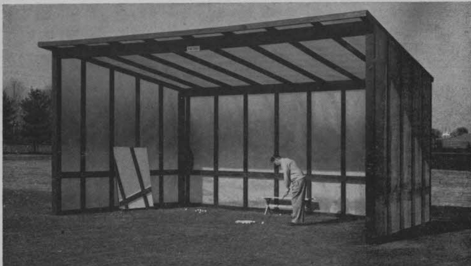
Bill Moran, professional, Concord CC, Wilmington, Del., practices under "shed" built for members who don't want the weather to interfere with their winter and early spring practice. Built of DuPont "Cel-O-Glass", a plastic coated wire mesh product, over wooden frame, the 24 ft. by 15 ft. structure although not completely transparent lets in plenty of light and heat but keeps out rain, wind and the cold. Idea for the new shed developed from a recent luncheon discussion by a group of Concord members headed by Grounds committee chairman F. S. Wilcox, Jr.
