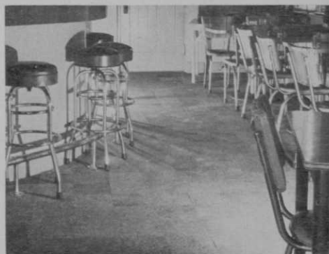
Installation of Do-All corded rubber floor tile.
