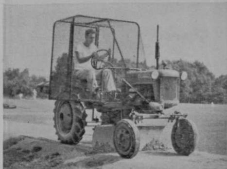
GRADES GROUND WITH DOZER BLADE
