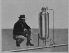
equipment fits any sprinkler system and completely eliminates the labor required to fertilize in the regular manner. The unit operates entirely by the movement of water in the sprinkler pipe line.
