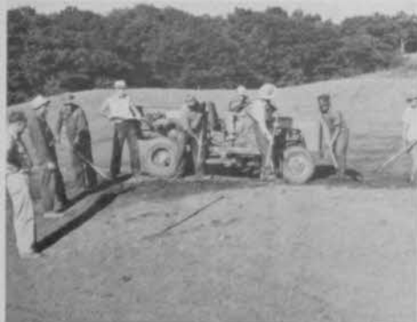
Preparatory to seeding the 4th green at North Oaks workmen rake stones and spread topsoil under the watchful eyes of Bill Fellows, agricultural engineer for Stanley Thompson and Associates, and George Hawkinson, foreman of the construction crew building the course.
