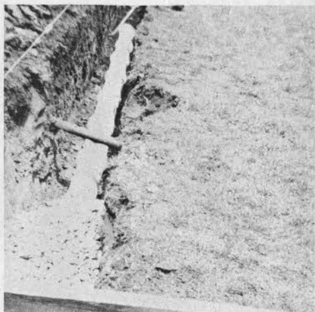
Stone backfill was put in as drain line was laid.
