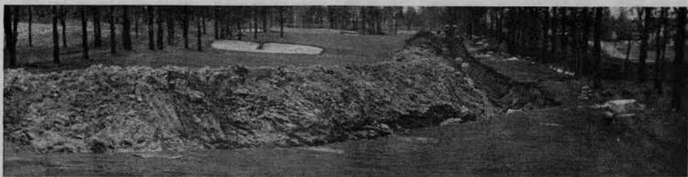
Main drain down 11th fairway. At close of 1949 season no signs of this major operation in digging were evident on the Beverly course.
