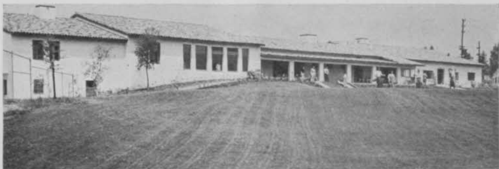
The beautiful new clubhouse at Rancho municipal golf course in Los Angeles, host course to the 24th annual U. S. Amateur Public Links Championship July 9-16, is decorated throughout in modern style. Clubhouse as well as course construction was financed from golf revenue, not taxes.
