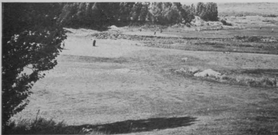
The laying of 4000 feet of tile and digging 14,000 feet of four-foot ditch has made possible the excellent green shown here in the low lying area on the new Butte course.
